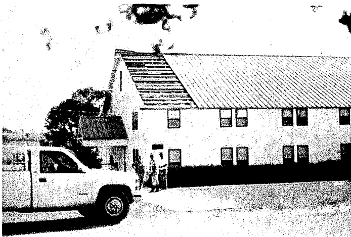
Parish Hall roof damage from the 2001 storm
