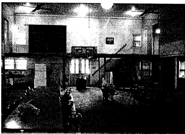
West end of the Parish Hall during the 1999 renovations
